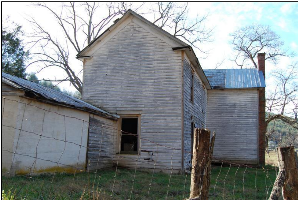
Figure 18: House [A] – south rear and west side elevations of main block and ell with stuccoed, concrete-block springhouse at left
