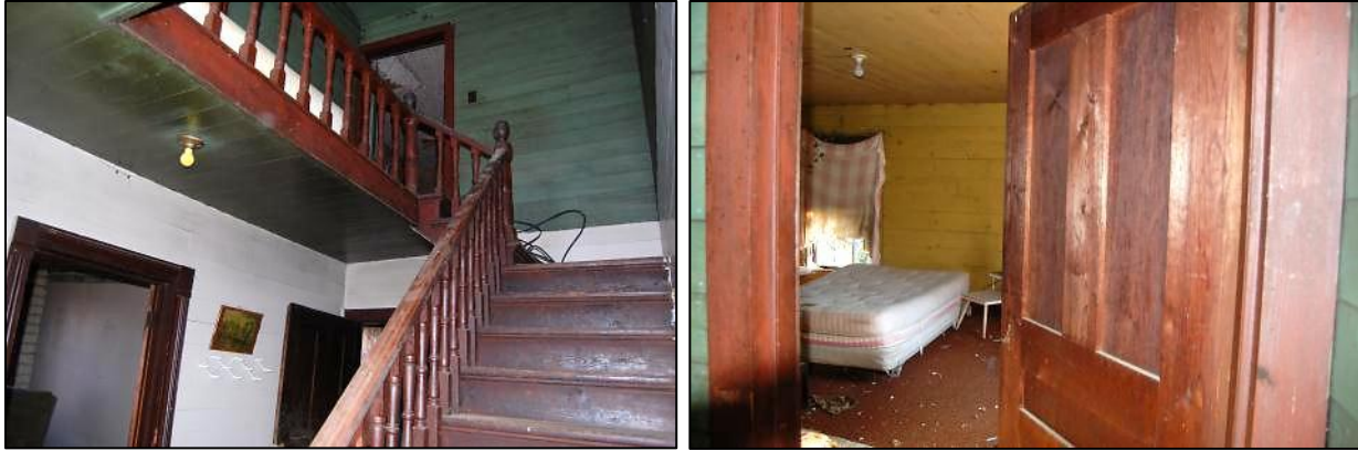
Figure 21: House [A] – stair hall at left; east upstairs bedroom at right
