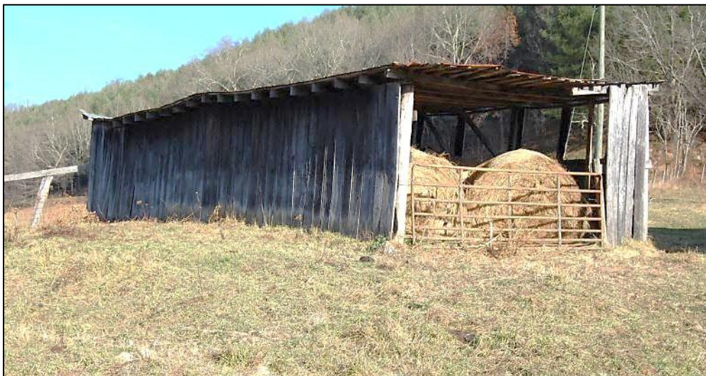
Figure 29: Shed [H] – looking north
