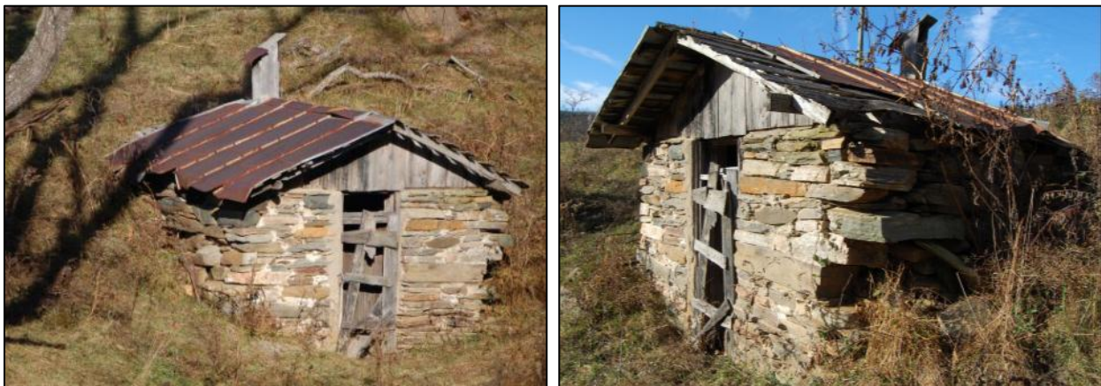
Figure 27: Cellar [F] – looking northwest, at left, and looking southwest, at right
