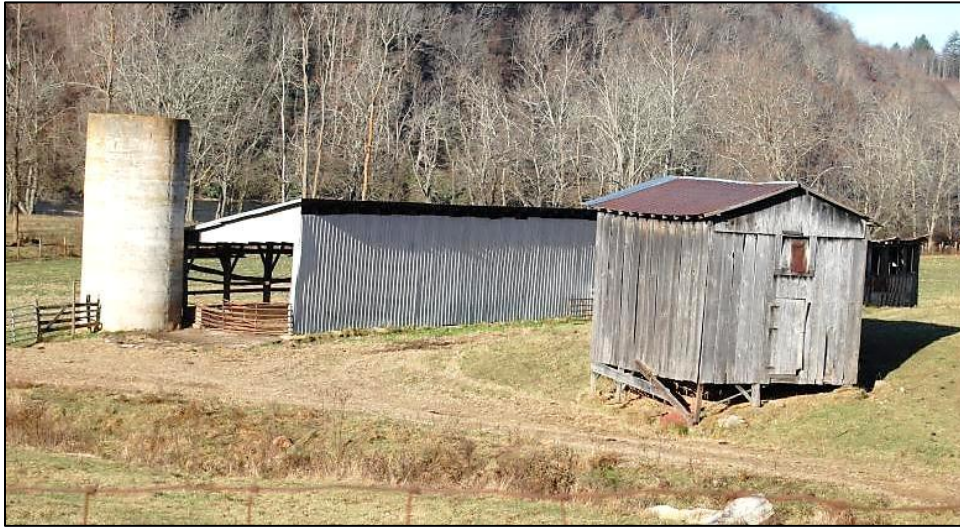
Figure 30: Pole barn [I] – looking southwest at pole barn [I] at center, silo [J] at left, granary [G] at right, and shed [H] at far right, with the New River in the background
