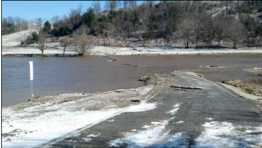
Figure 56: Looking northeast from Farmers Fish Camp toward Gambill Family Farm, ca. February 1, 2013; caption reads “This was a low water bridge over the New River that normally goes under water during high water events in Alleghany County north of Sparta.” (source: http://www.flickr.com/search/?q=%22farmers%20fish%20camp%22%20road%20bridge and NCDOT communications)
