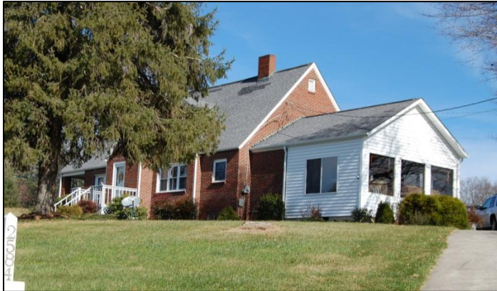
Figure 60: Johnsie Gambill McIntyre House, east front and south side elevations, with modern vinyl-sided addition
