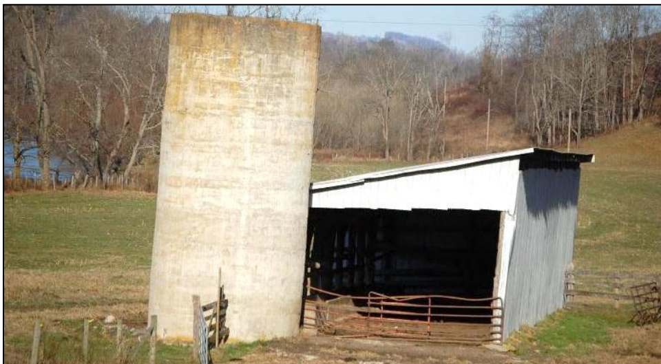
Figure 31: Silo [J] – looking west at silo [J] at left and pole barn [I] at right with New River in background
