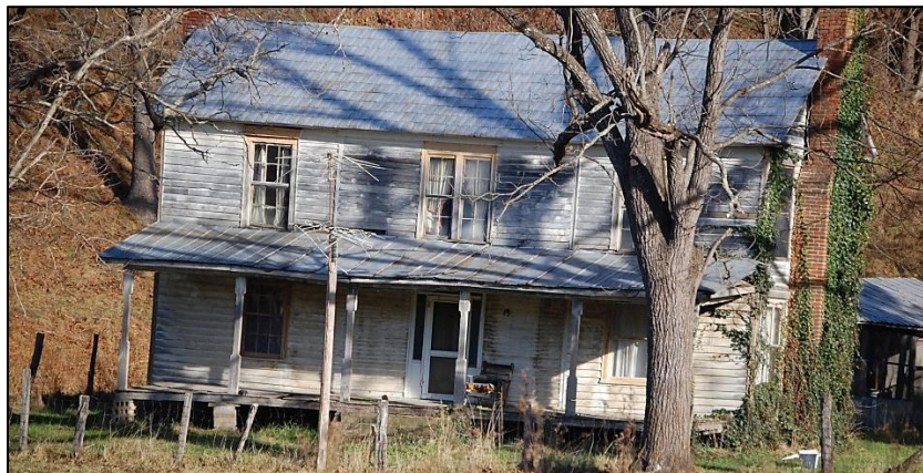
Figure 8: South front elevation of House [A] at Gambill Family Farm
