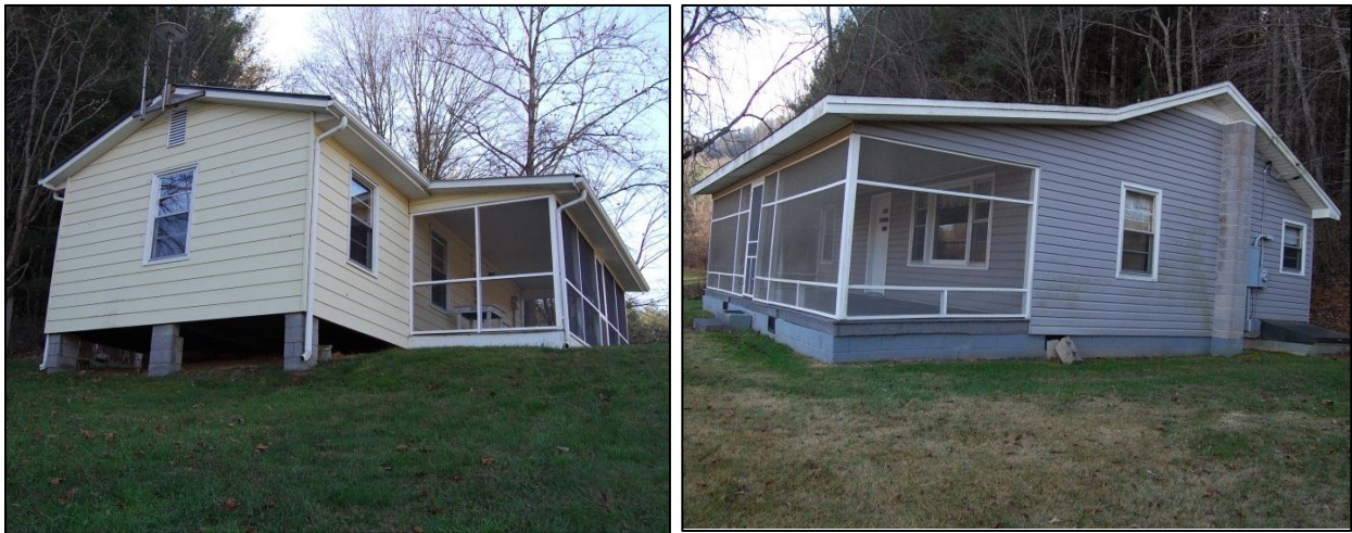
Figure 49: North front and east side elevation of 1350 Farmers Fish Camp Road, at left; east front and north side elevations of 1364 Farmers Fish Camp Road, at right
