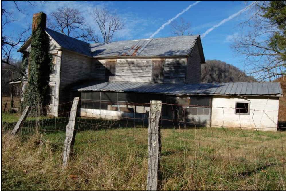
Figure 19: House [A] – east side and south rear elevations of main block and ell with screened porch and springhouse at center and right
