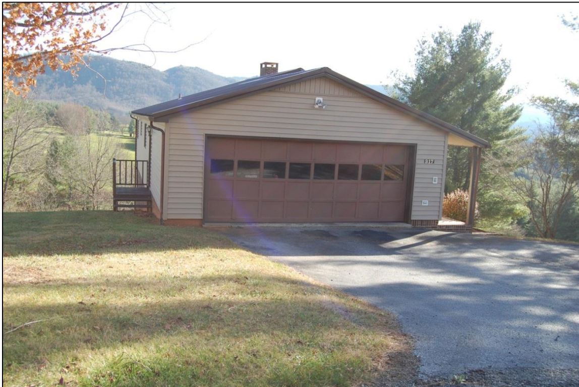
Figure 87: View within potential Farmers Fish Camp Road/New River rural historic district of modern house on south side of Buckeye Ridge Road with New River Country Club to rear
