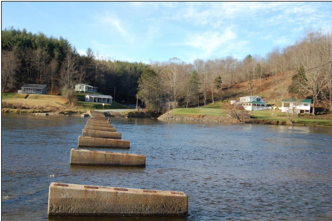
Figure 69: View within potential Farmers Fish Camp Road/New River rural historic district of pilings of Bridge 265, Farmers Fish Camp at right, Muncy Steadham House at center left, and later houses at far left
