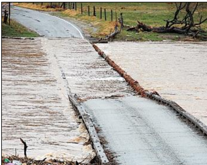
Figure 55: Farmers Fish Camp Road bridge, intact during flooding as it functions as a low water bridge (source: Alleghany News , n.d. and http://www.alleghanynews.com/archive/122_31/Flood%203.jpg )
