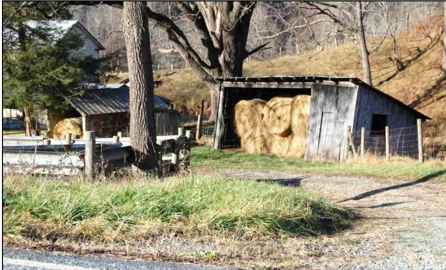
Figure 26: Tractor shed [E] – looking southwest from Farmers Fish Camp Road at tractor shed [E] at right, privy [D] and garage [C] at center left, and ell of house [A] at far left
